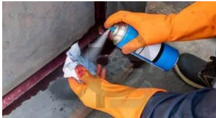
Fig. 5 Clean with cleaner- The solvent should be sprayed onto the cloth, which once soaked should be used to clean the surface
